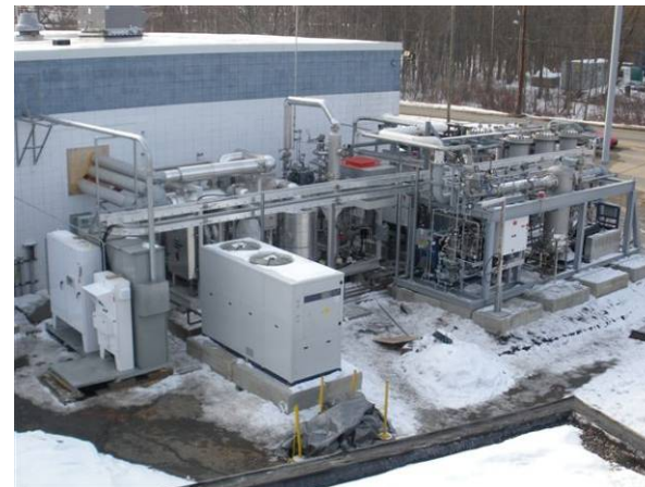
Anode Exhaust Processing and H 2 PSA
