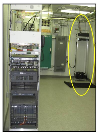
Station Battery Stack with Fuel Cell
