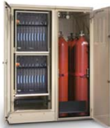
4,000 Watt - 48 kWh Configuration
