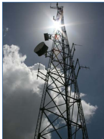
Hydrogen fuel cells providing critical backup power
