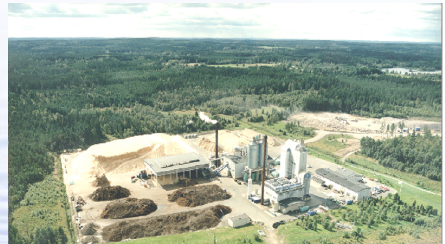
Varnamo Sweden, 100 mt/day, 6 MWe + 9 MWth demo run for 5 years, now being retrofitted for BTL
