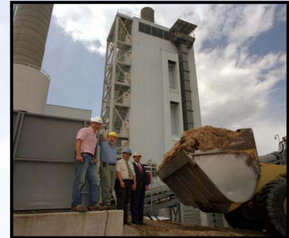
300 ton/day gasifier Burlington Electric, VT
