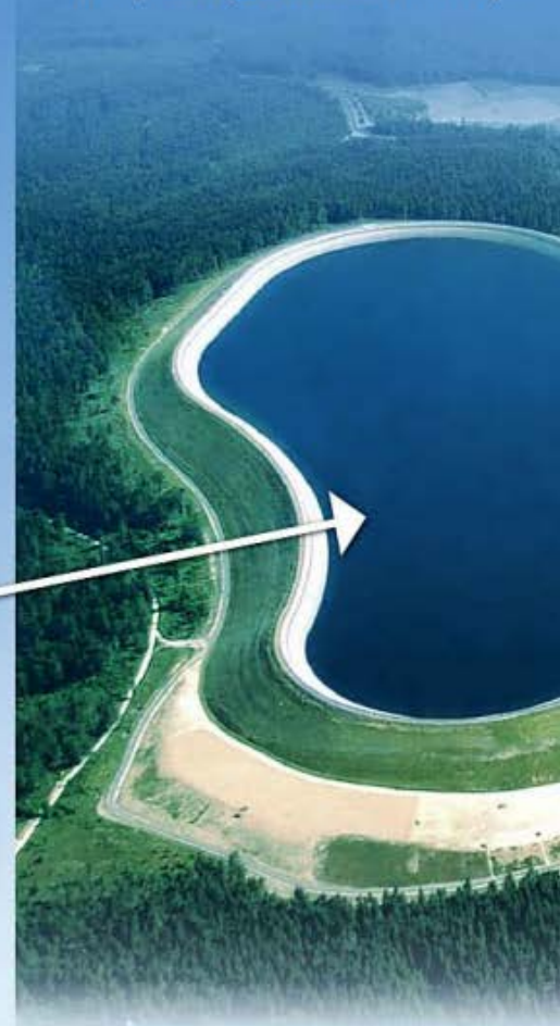
Pump storage Goldisthal, Thüringen
