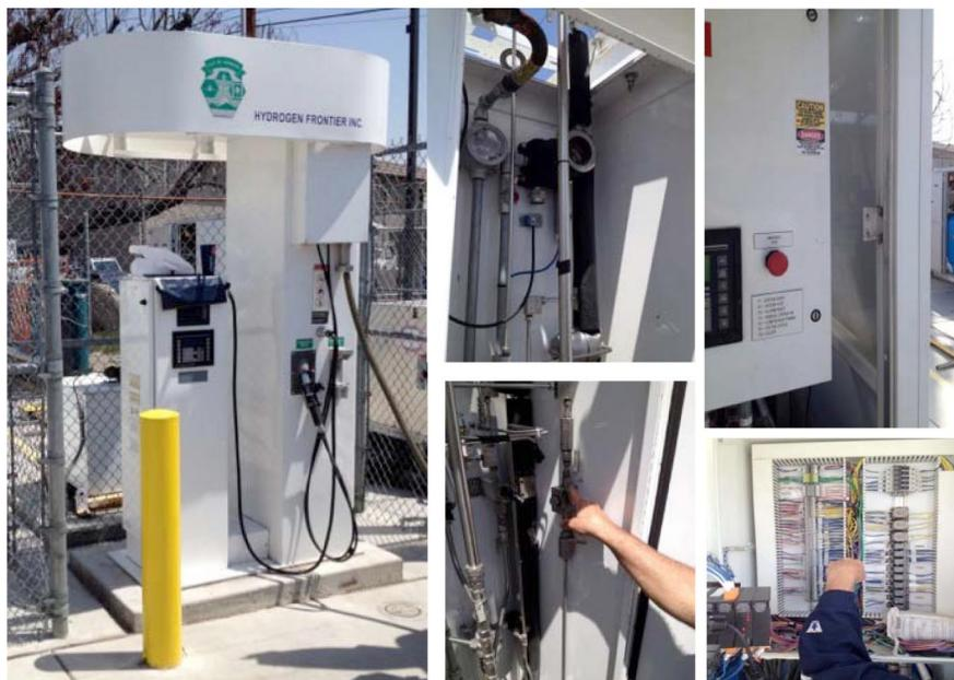
**FIGURE 2.** Photographs taken on site at the Burbank Hydrogen Frontier location. Although four suitable locations were identified, the location inside the hydrogen dispensing island enclosure (left and top/bottom center) was deemed the most desirable for single sensor unit deployment. Locations for test units to access 24-V direct current power were also identified (lower right).
