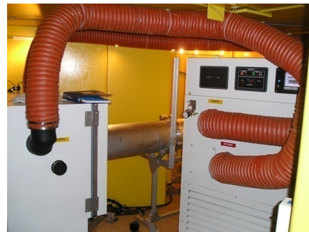
Freeze Chamber Installed inside the Imaging Facility
