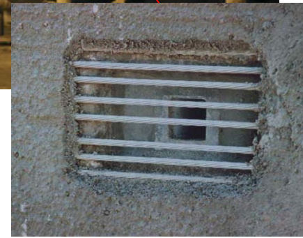
Winding and tensioning of steel tendons
