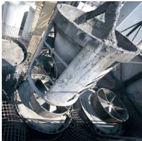
Casting of a concrete core around the steel cylinder
