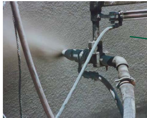
Shotcrete application for corrosion prevention
