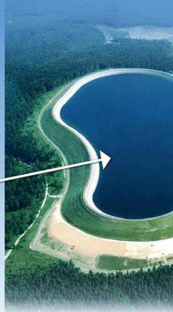
Pump storage Goldisthal, Thüringen
