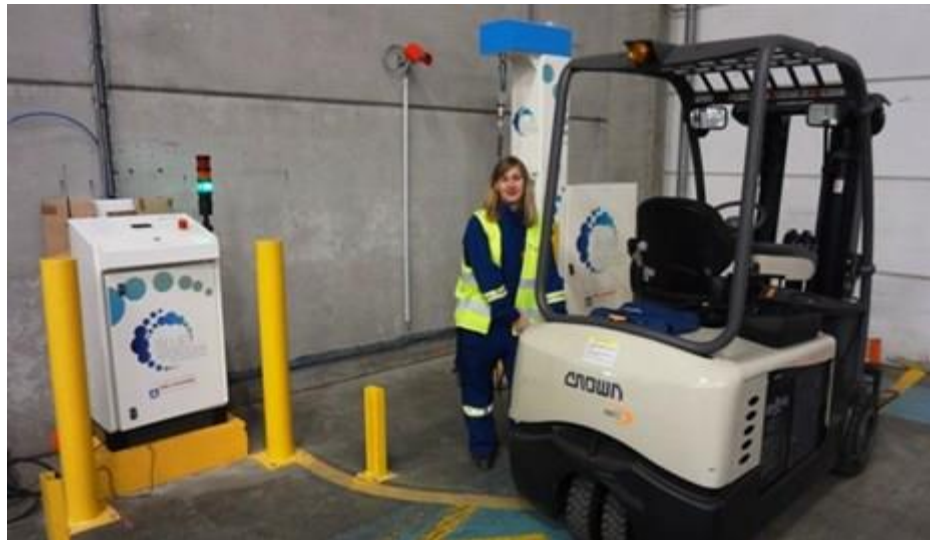
Figure 7. Hydrogen fueling for material handling equipment
