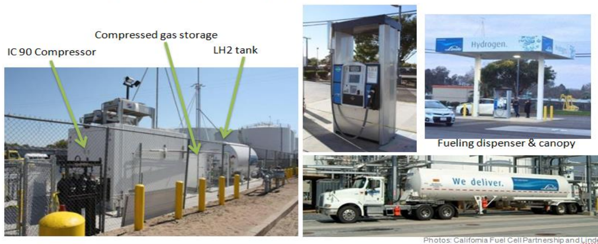
Figure 3. Delivered hydrogen station (liquid delivery example)
