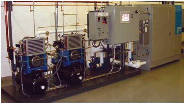
FIGURE 4. Installed StarCell™ System, July 2005
