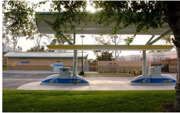
FIGURE 3. Infrastructure, Chino Station
