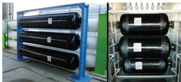
FIGURE 4. Three-Bank Hydrogen Cascade Using Composite Pressure Vessels
