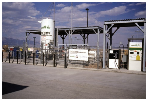
FIGURE 3. View of the Fuel Station
