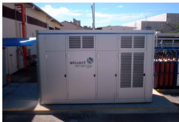
Figure 3. Stuart Power Park Electrolyzer at the HFCTF
