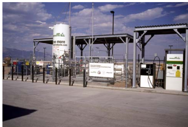
Figure 3. View of the Fuel Station
