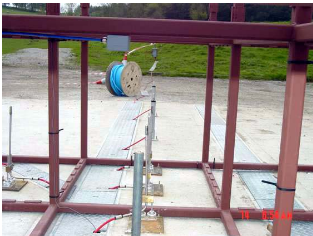
Figure 3. Testing Sensors with Igniter
