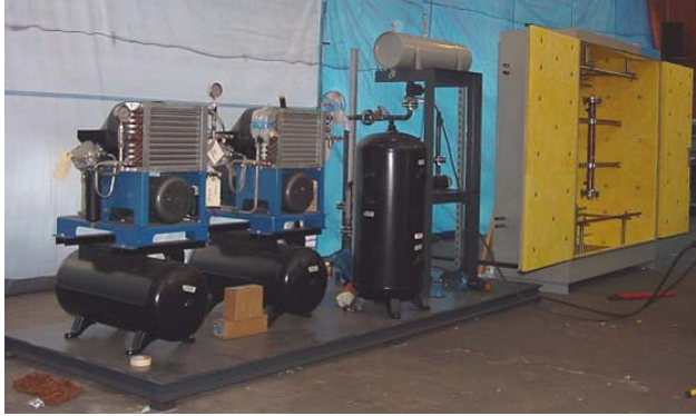
Figure 2. StarCell Construction, April 2005
