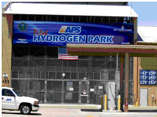
Figure 1. APS Pilot Hydrogen Park in Downtown Phoenix (The park is open to the public for motor vehicle fueling.)
