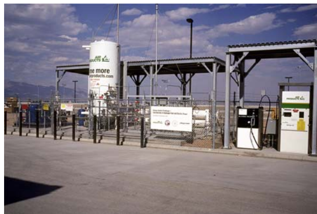
Figure 3. View of the Fuel Station
