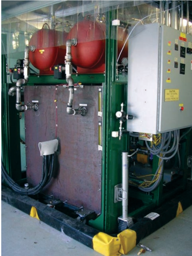
FIGURE 1. Ambient Pressure Plastic Electrolyzer stack
