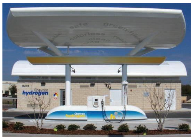
FIGURE 1. Infrastructure at the Orlando Station
