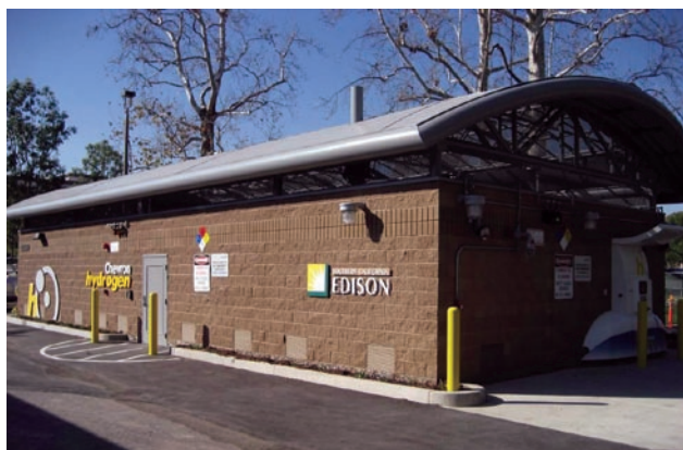
FIGURE 2. Infrastructure at the Rosemead Station
