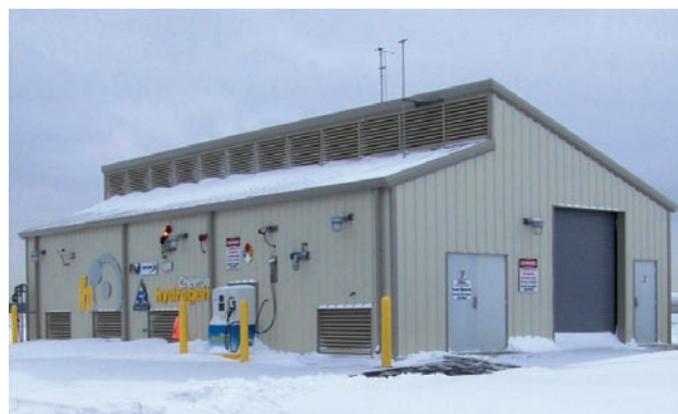
FIGURE 1. Infrastructure Selfridge Station
