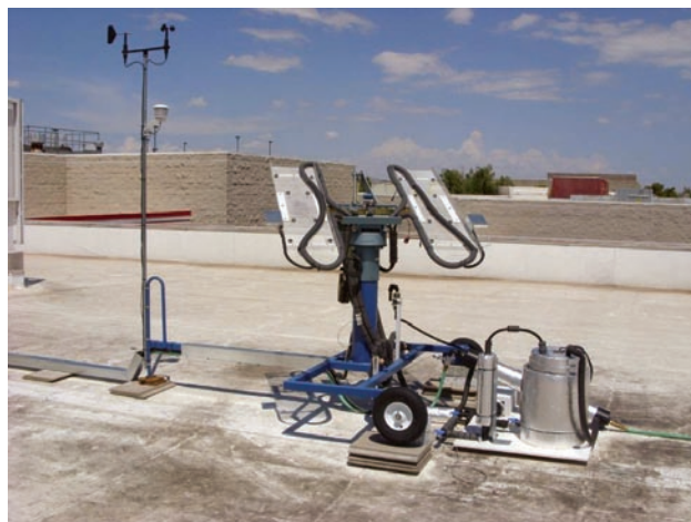
FIGURE 2. On-Sun Testing Facility Installed on Roof of UNLV Building
