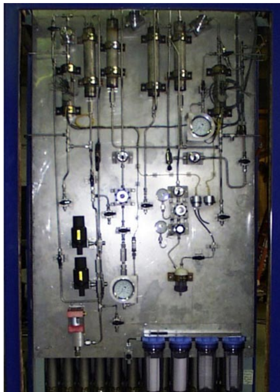
FIGURE 4. Valve Control Panel Fabrication in Progress
