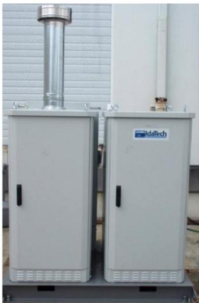
IdaTech 5kW<sub>net</sub> indirect methanol fuel cell
