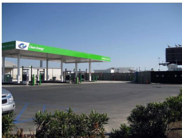
FIGURE 2. Clean Energy Station near LAX in Los Angeles, CA
