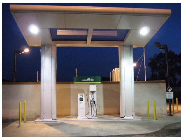
FIGURE 1. UCI 350/700 Bar Gaseous Hydrogen Dispenser
