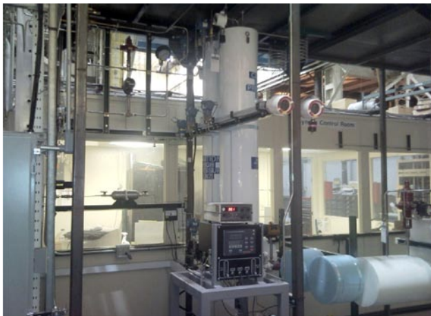
FIGURE 2. Pilot-Scale Test System
