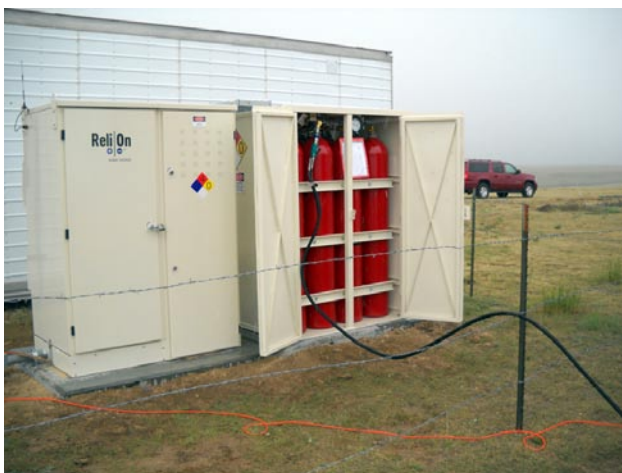
FIGURE 2. Completed AT&T Site (Byers, CO) Undergoing Initial Fill of the HSM
