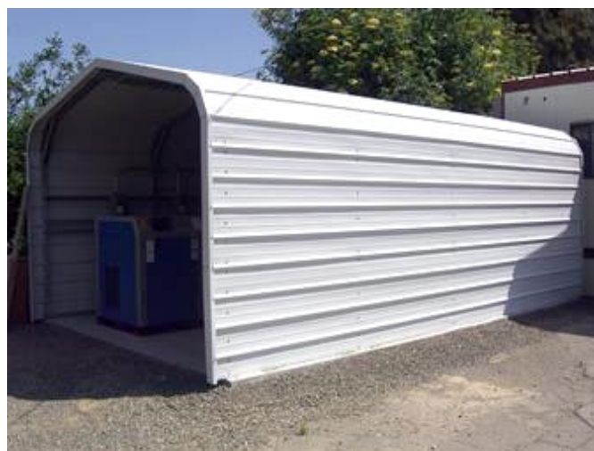
FIGURE 1. Constructed Outdoor Test Shelter at UC Davis
