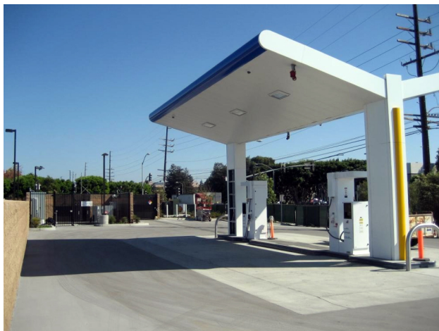
FIGURE 5. The Dispenser Area at Shell's Torrance, California, Fueling Station, which is Supplied by an Air Products Pipeline
