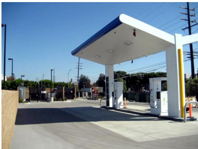
FIGURE 2. Torrance, CA Hydrogen Pipeline Fueling Station
