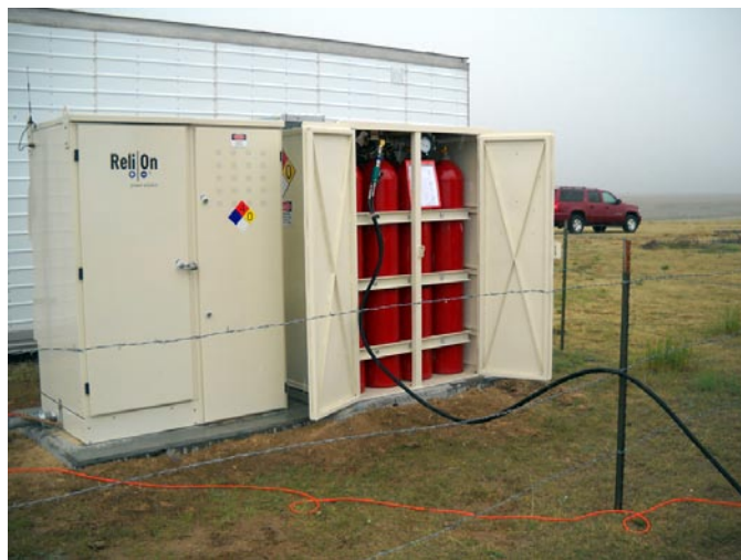
FIGURE 2. Fueling of HSM at Completed AT&T Site in CO
