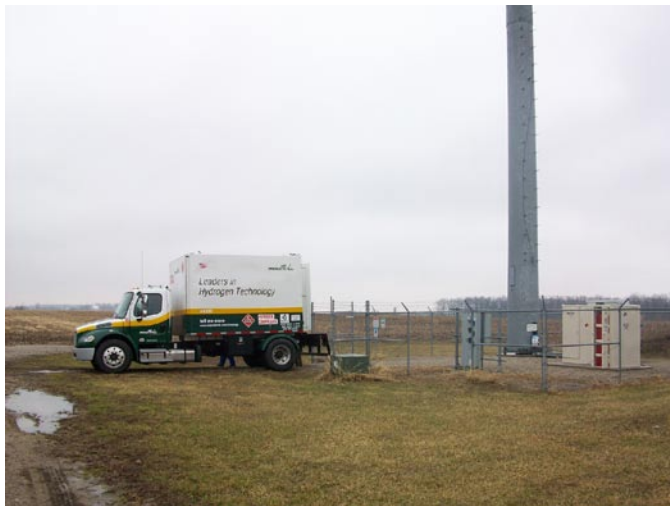
FIGURE 1. Completed AT&T Site in MI Showing 'Straight Truck'
