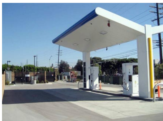
FIGURE 3. The dispenser area at Shell's Torrance, California, fueling station, which is supplied by an Air Products pipeline
