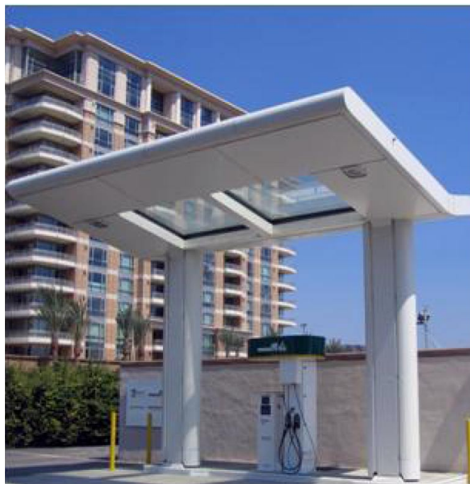
FIGURE 1. UCI 350/700 Bar Hydrogen Fueling Station
