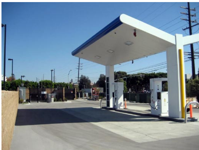
FIGURE 2. Torrance, CA Hydrogen Pipeline Fueling Station
