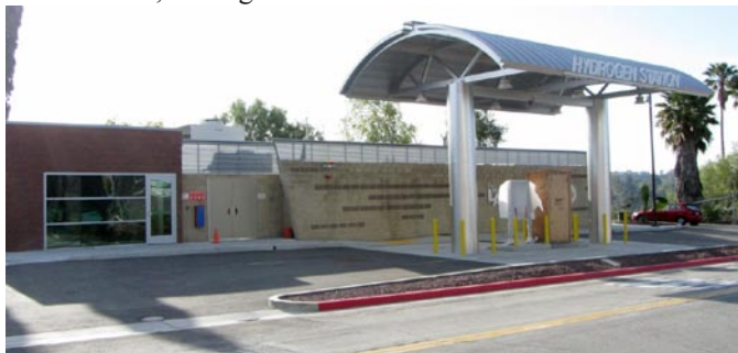
FIGURE 1. CSULA Hydrogen Fueling Facility
