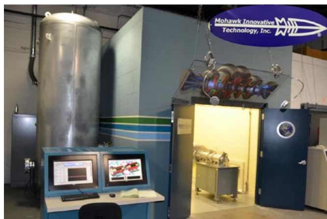
FIGURE 1. Dedicated MiTi ® test cell, 200-kW single-stage compressor and closed-loop gas system.
