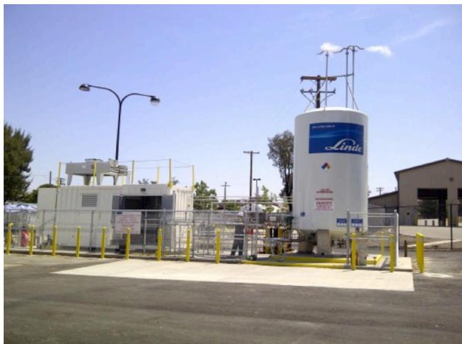
**FIGURE 1.** Liquid Hydrogen Pump Installed at the LLNL Campus
