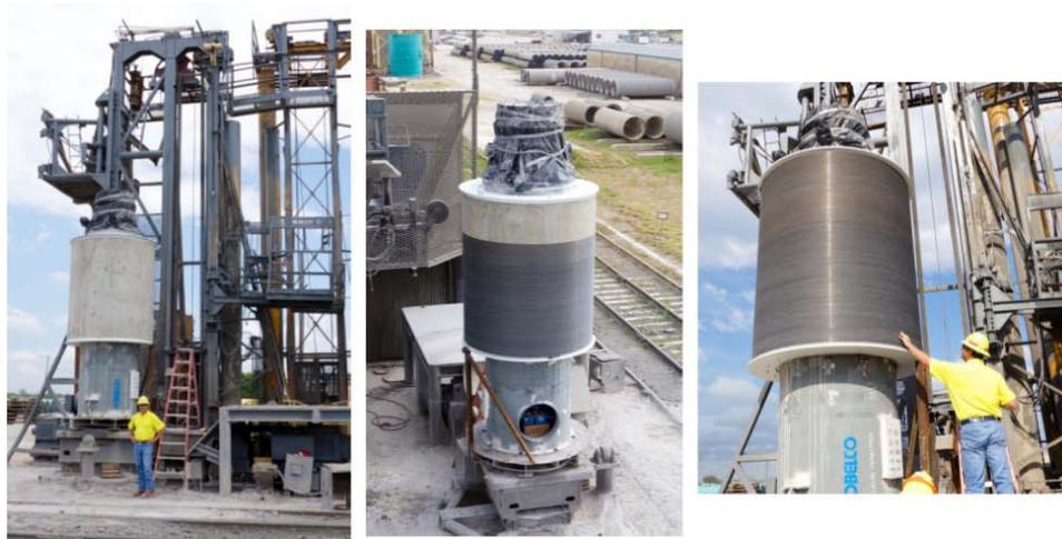
**FIGURE 3.** Wire wrapping during SCCV construction
