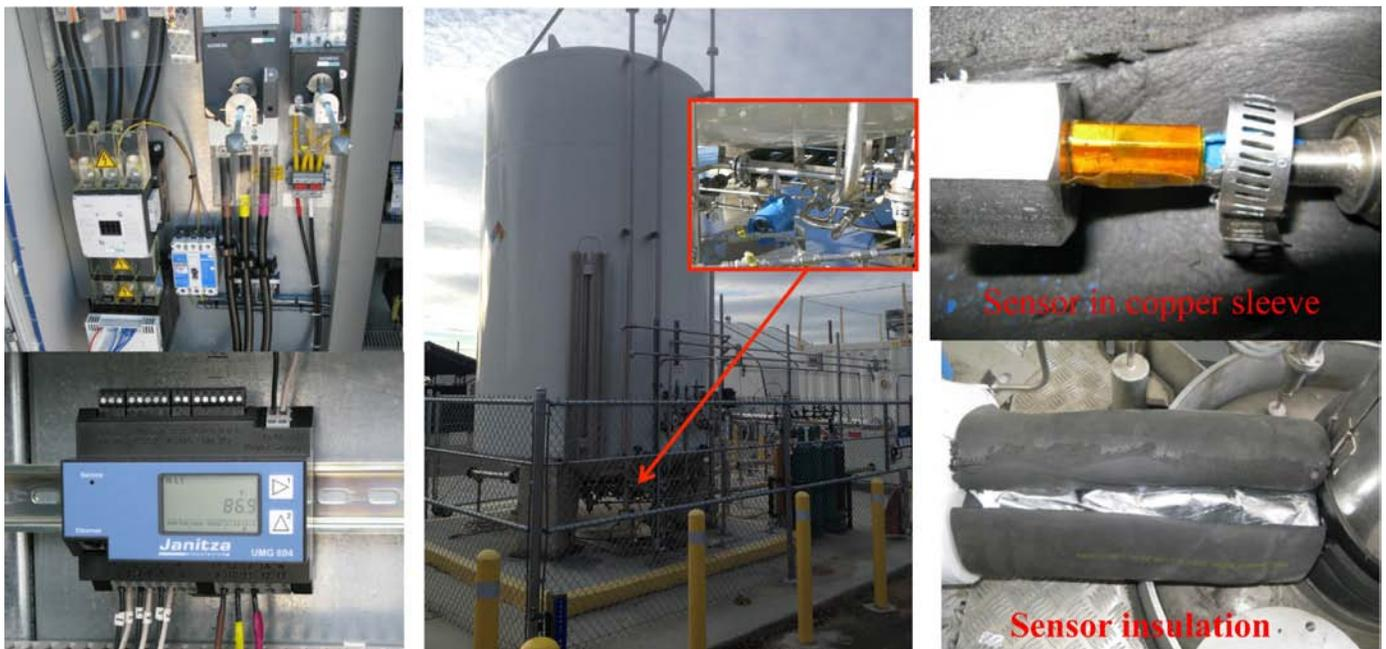
**FIGURE 4.** New instrumentation installed on the liquid hydrogen pump including (a) power analyzer, (b) vent line mass flow meter, and (c) temperature sensor at the pump outlet
