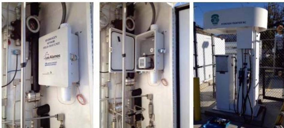
**FIGURE 1.** (Left) Sensor unit installed inside dispensing island with cover closed. (Center) Cover open showing wireless transmitter and sensor and metal shielded power supply. (Right) Completed installation with dispenser unit enclosure sealed and ready for service.
