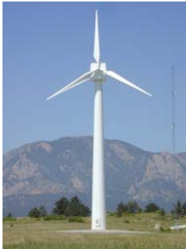
Northern Power wind turbine
