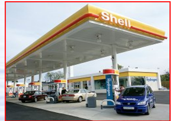
Washington, DC Hydrogen Fueling Station
