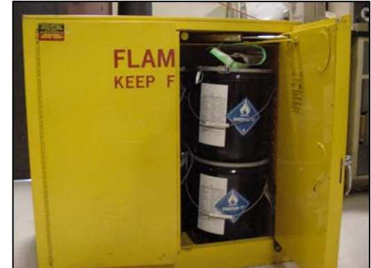
Incoming material stored in fire cabinet
