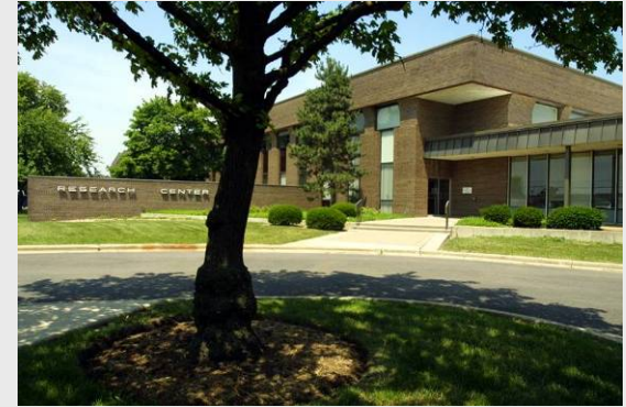
GTI's Main Research Facility
