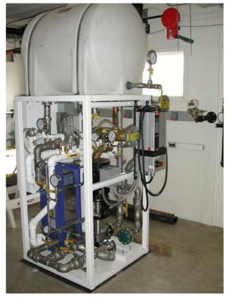
100-kW cooling system being installed in the Fuel Cell Test Facility
