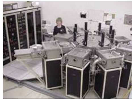
cluster tool installation
