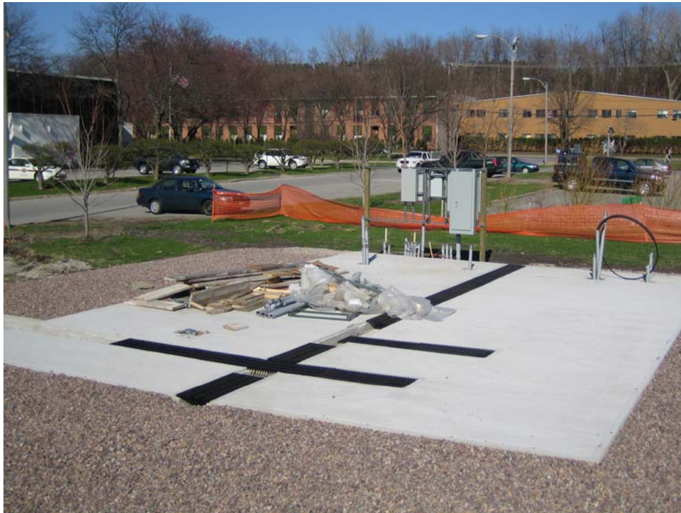
Fueling Station Site April 2006 at Burlington (VT) Department of Public Works
